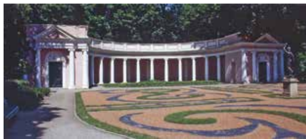
210. Neo-classical colonnaded entryway into the Oleksandriya Park, Bila Tserkva, late 18th century.
