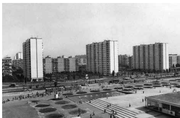
215. Apartment complex in the Soviet functional Constructivist style, Obolon District, Kyiv, 1980s.
