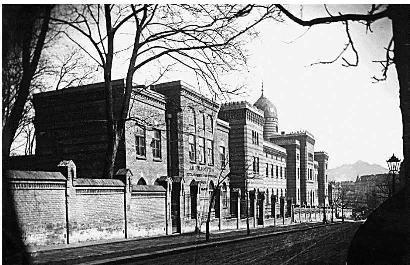
Fig. 11. The Israelite Hospital, view from southwest, the ambulatory is seen on the left, photograph ca. 1914. Lviv Historical Museum.
