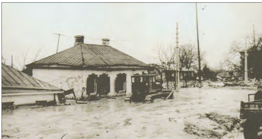
Residential buildings on Frunze Street flooded to the ceilings and windows.
