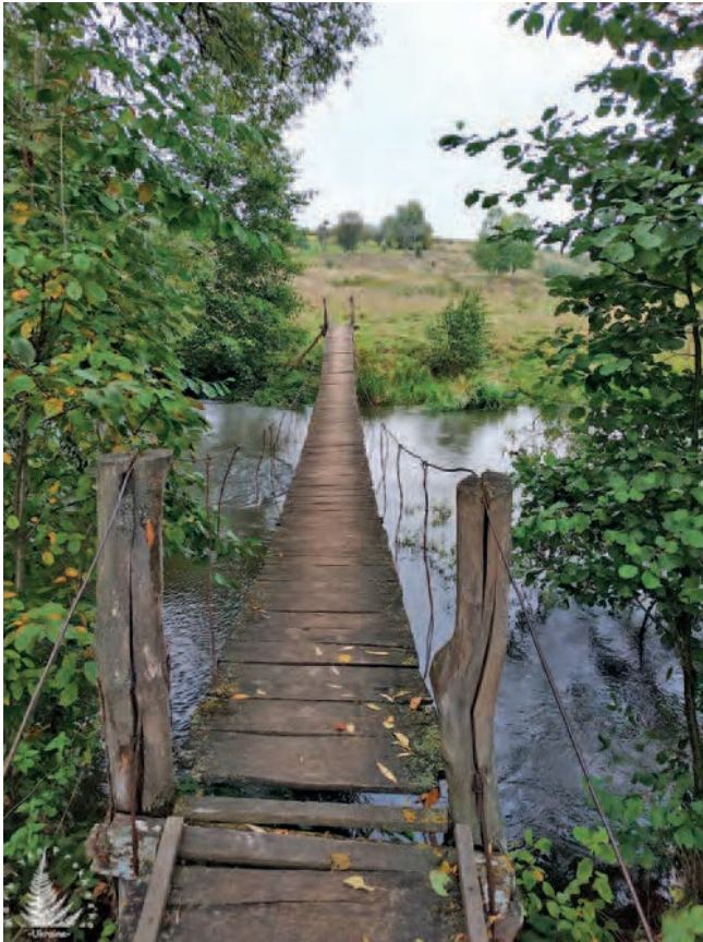
Bridge for observing time.
